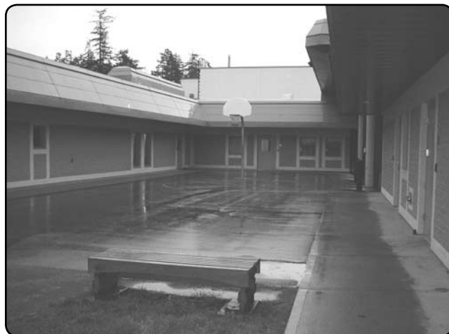
Art room in custody centre (top); mural painted by youth (middle); and courtyard (bottom).
