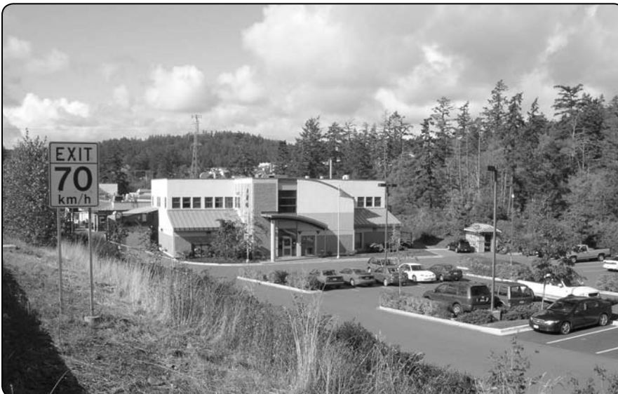
Entrance to a custody centre.
